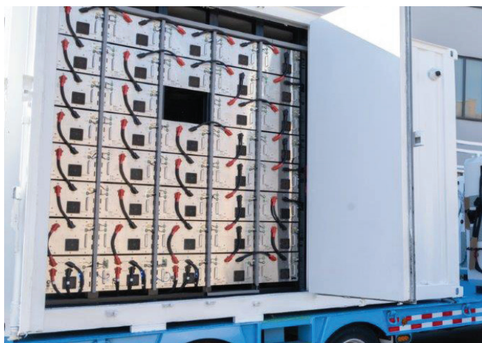
PICTURED: PROMIS non-walkable battery room
