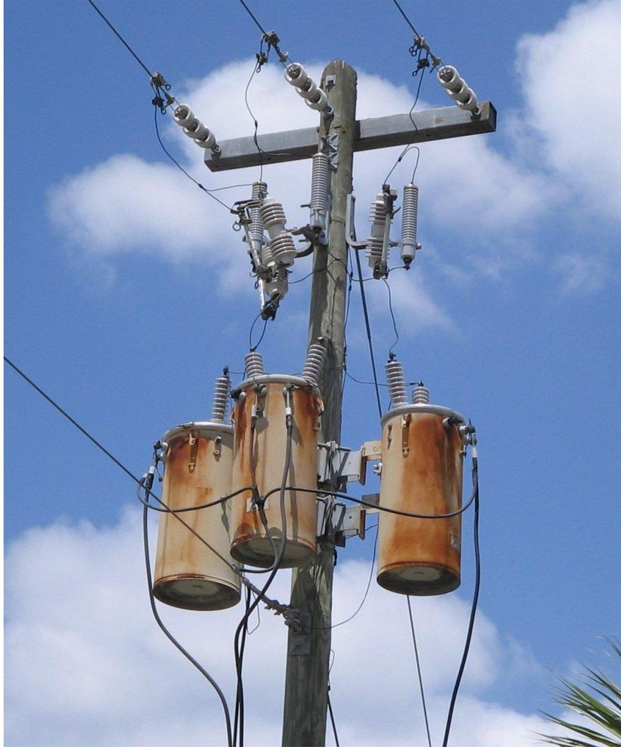
**Figure 3** A bank of service transformers does not look new, because they aren't, but they are good to go in a system that is trying to get the most from its past investments in equipment. The utility's challenge is to separate these units, which can be expected to give satisfactory service for many years to come, from other units that won't.
